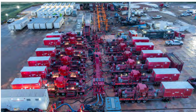
Electric fracturing operations
